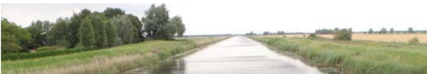
The Middle Level Main Drain at Neeps Bridge
